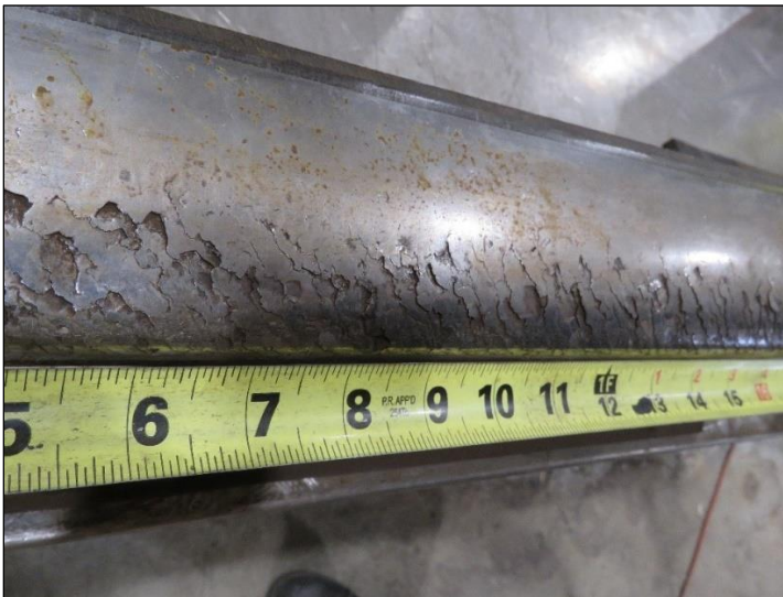
Figure 6. Condition of running surface of the rail head recovered at the occurrence site (Source: Canadian Pacific Railway)
