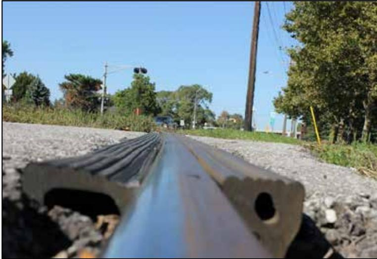
Figure 19. A style of displaceable reduced flangeway gap filler currently in use in the United States (Source: Polycorp)
