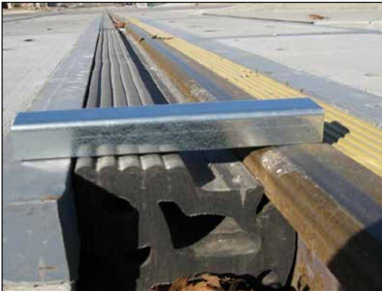
To date, flangeway gap fillers in North America have been used primarily for light rail transit systems or commercial purposes. Two Class I railways are using flangeway gap fillers in specific applications.<sup>33</sup> Some European railways are using a displaceable flangeway gap product designed for temperatures as low as  $-25^{\circ}\text{C}$  and for train speeds of up to 120 km/h that also
