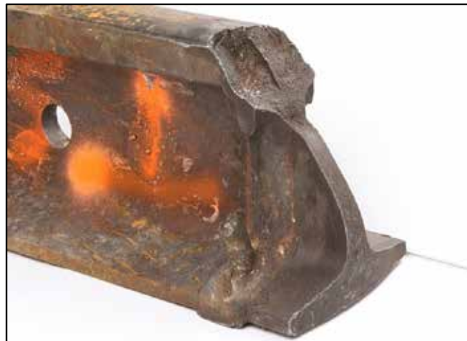
Figure 15. Photograph of thermite weld on the east end of the removed parent rail with vertical split head defect in the rail head
