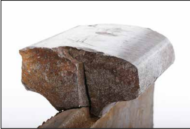
Figure 17. View of vertical split head in fragment of recovered 4-inch-long section of the east parent rail head
