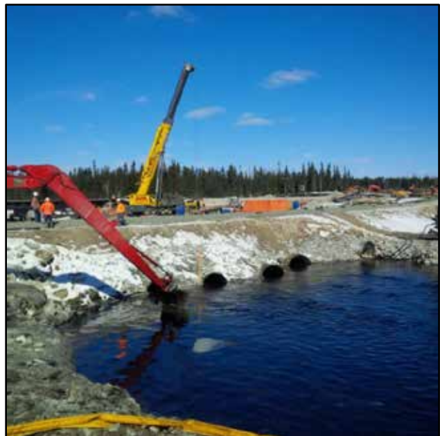
Figure 10. Diversion track over Makami River
