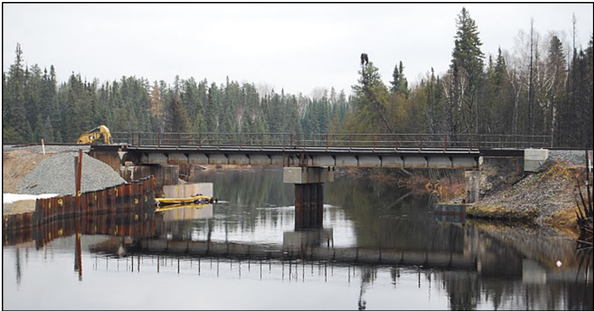
Figure 11. Replacement bridge over Makami River
