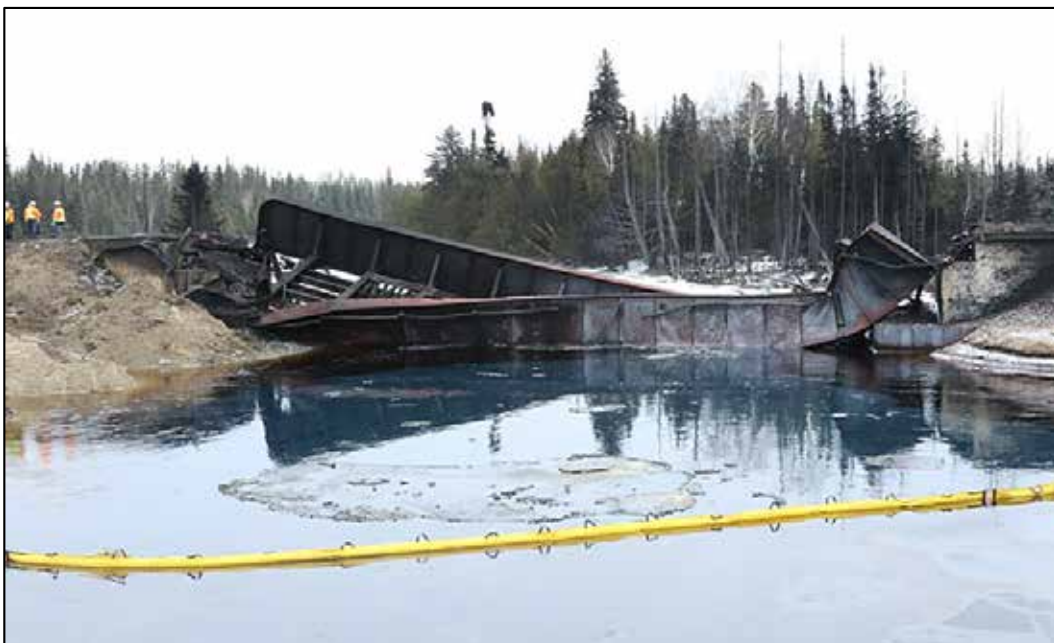
Figure 4. Bridge over the Makami River
