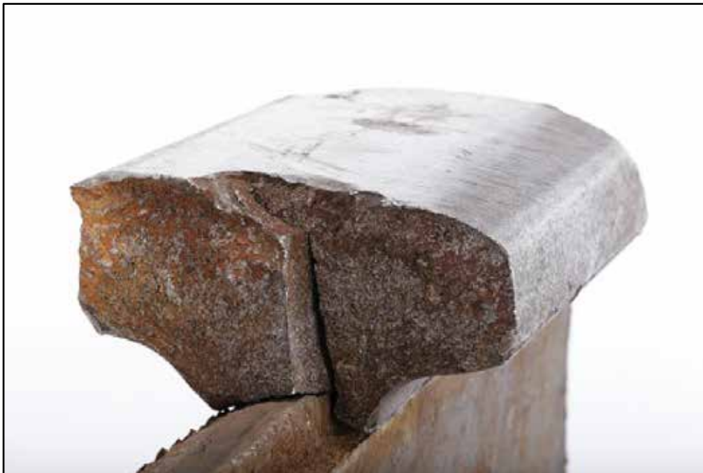
Figure 8. Gauge-side view of vertical split head defect in fragment of recovered parent rail head
