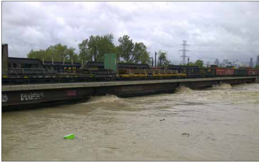
Photo 5. Bonnybrook Bridge (from upstream) on 21 June, at the height of the flood (Source: CP)
