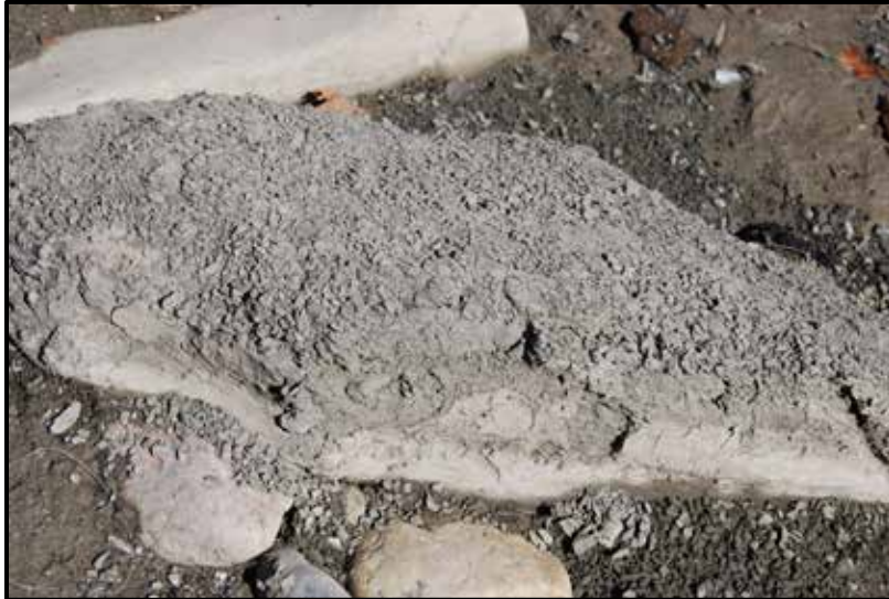
Photo 3. Broken piece of shale/sandstone similar to the bridge foundation
