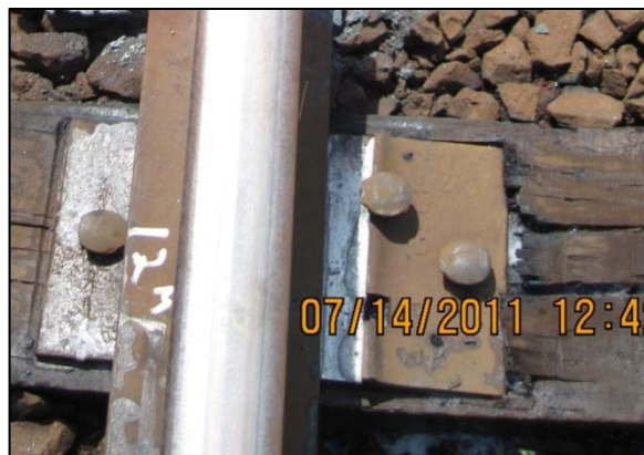
Photo 3c. Close-up showing old anchor cut on tie and tie plate plus more recent vertical/horizontal polishing on the anchor face
