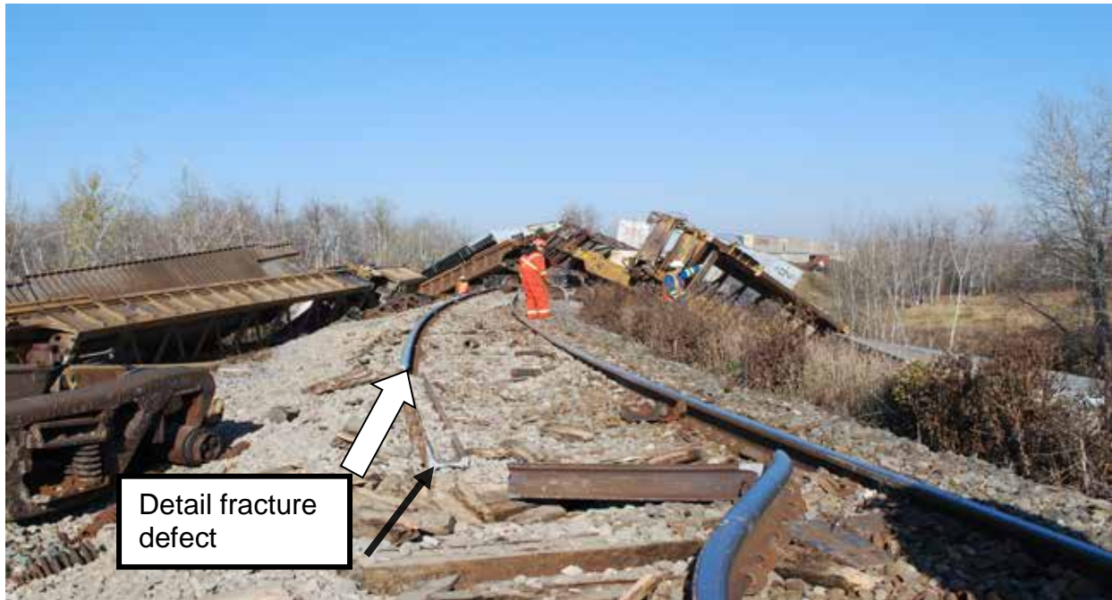
Photo 1. Derailed site looking north. (Note: Detail fracture defect in rail end)
