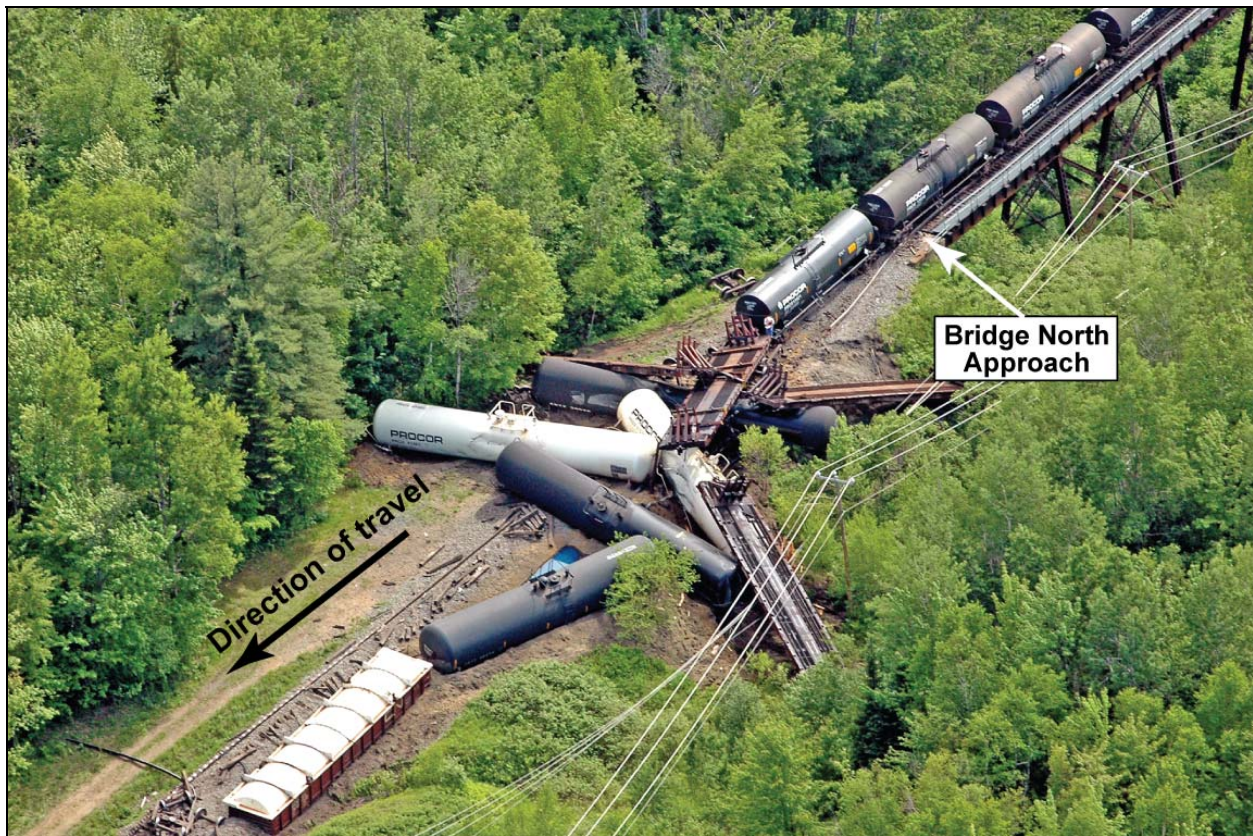
Photo 1. Accident site (Source: Newspaper Le Nouvelliste )
