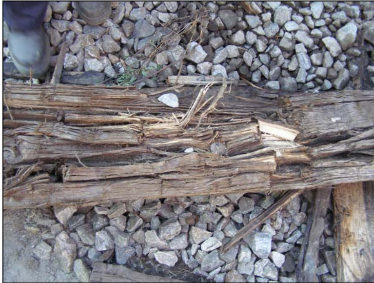
Photo 2. Track tie from the north approach
