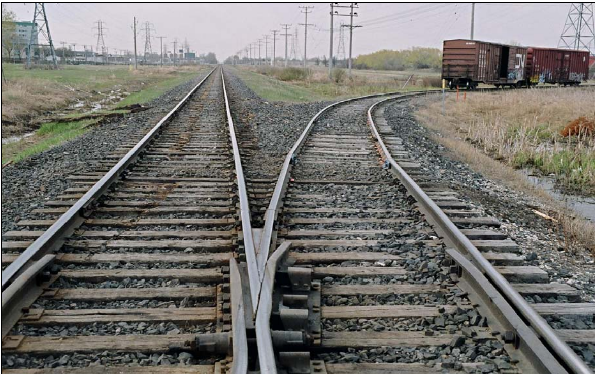
Photo 1. Turnout WC20 at Mile 1.8
