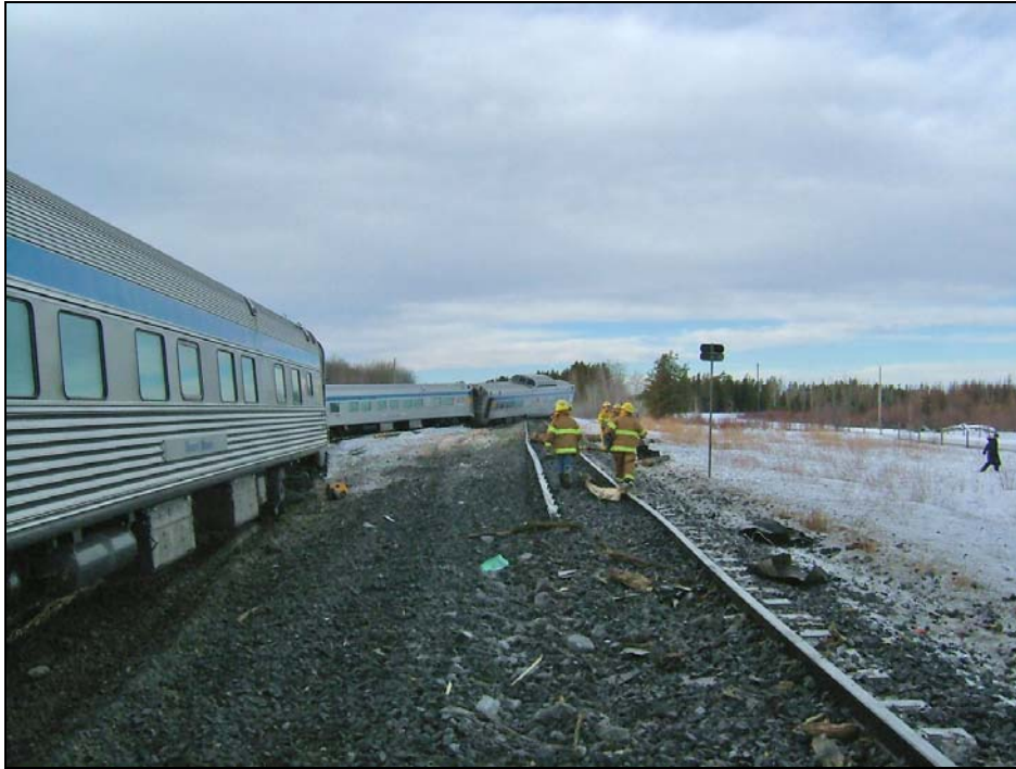
Photo 2. View of the derailment and associated track damage looking eastward from the crossing
