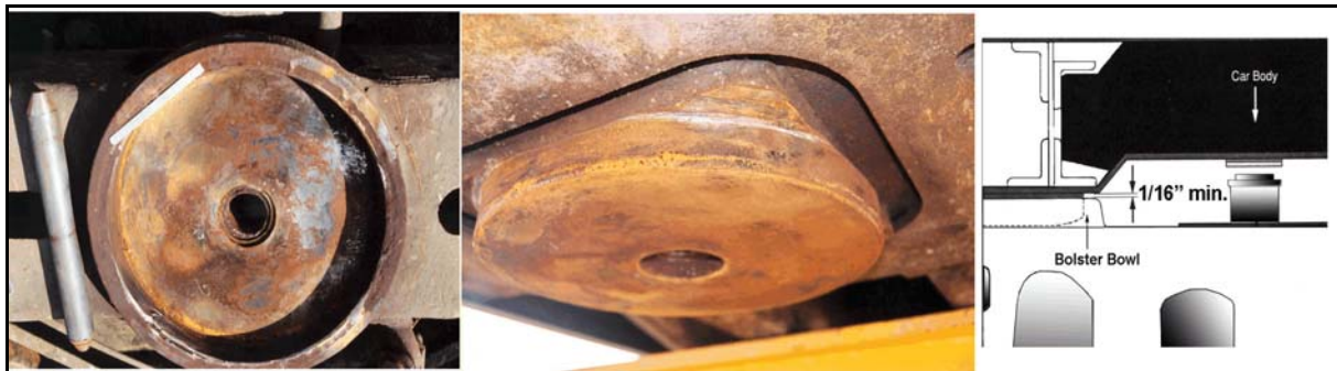
Photo 2. The truck bolster rim on car FURX 818699 was worn at four locations. The wear on the corners of the matching car body centre plate corresponded to the bolster rim wear. The sketch indicates the clearance between the two.
