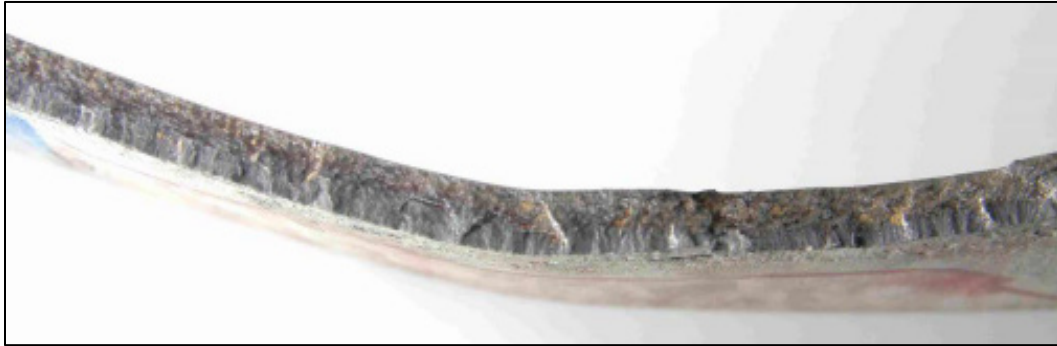
Figure 8. Interacting cracks shown on a portion of section 1 of the ruptured pipe (Source: Acuren)
