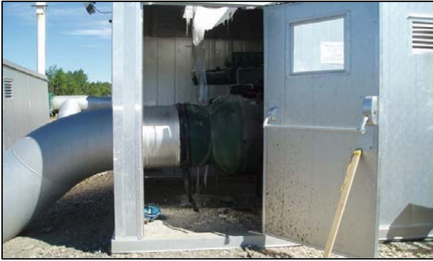
Photo 2. Egress door for MOV-0409 enclosure
