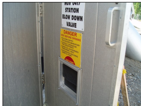
Photo 5. Air-quality testing port and associated signage
