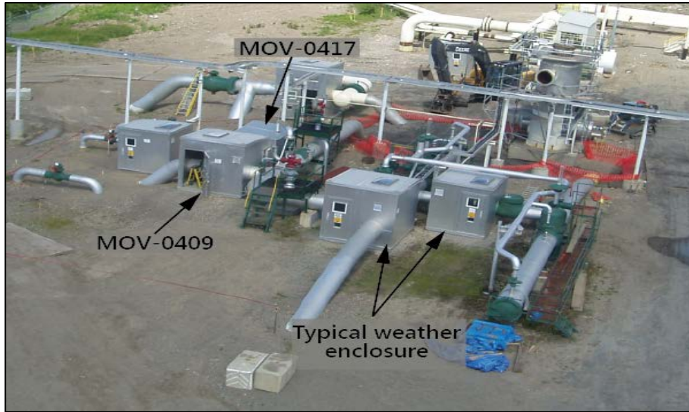
Figure 2. Aerial view of weather enclosure structures
