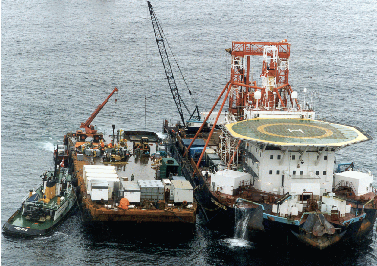
Figure 18: Heavy lift operation
