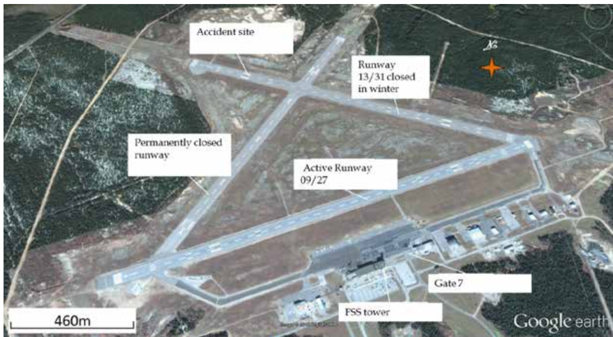
Figure 6. View of the Sept-Îles Airport (Source: Google Earth, with TSB annotations)
