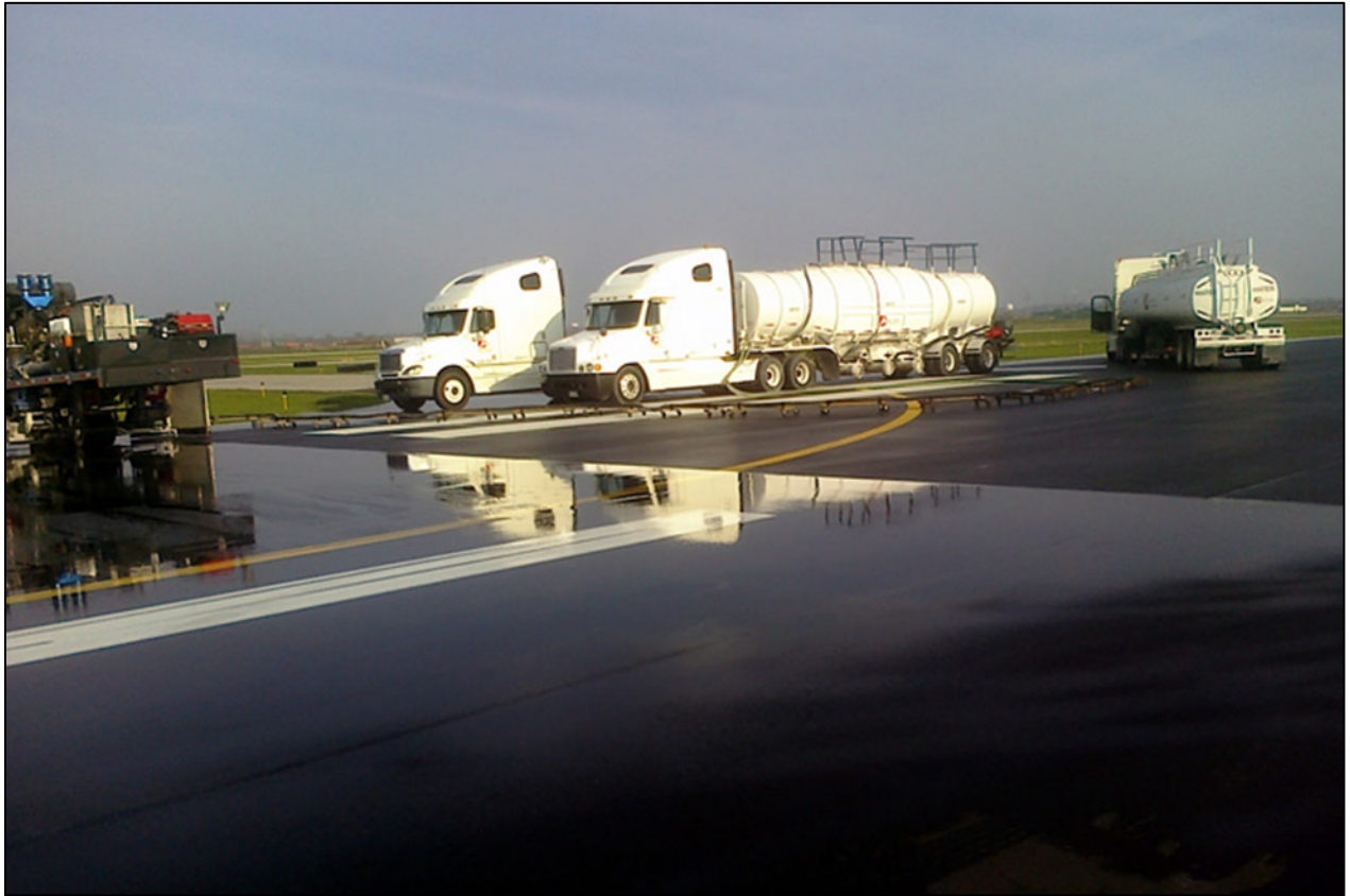
Photo 7. A grooved runway (the section where the trucks are parked) versus a non-grooved runway, shown after being flushed with water during the grooving process (photo used with permission from the St. Louis Downtown Airport [KCPS])
