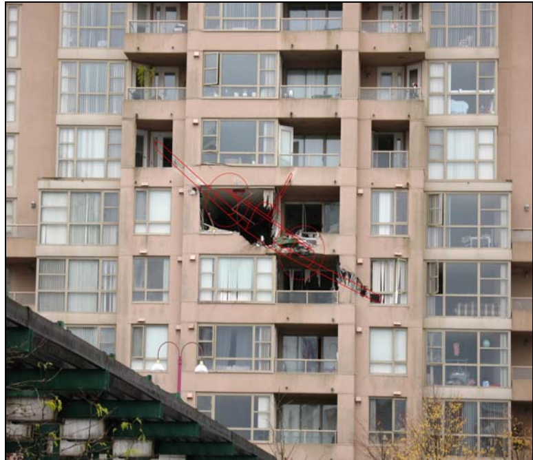
Photo 1. Impact damage
