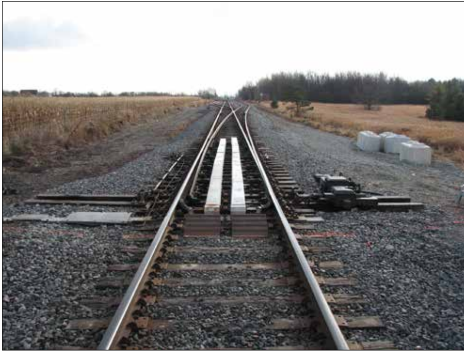
Photo 5. North turnout at Teston siding in Vaughan, Ontario
