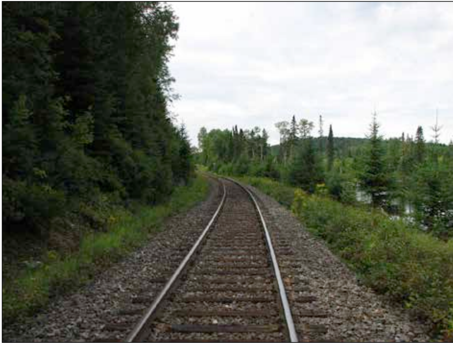
Photo 2. Railway right-of-way in the curve, at the north switch approach
