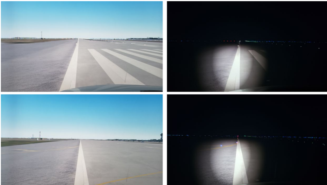
Figure 14. Simulated runway environments at the runway's left edge. Clockwise, from top left: daytime, at runway threshold; nighttime with reduced visibility, at runway threshold; nighttime, in displaced threshold area; daytime, in displaced threshold area. (Source: TSB)
